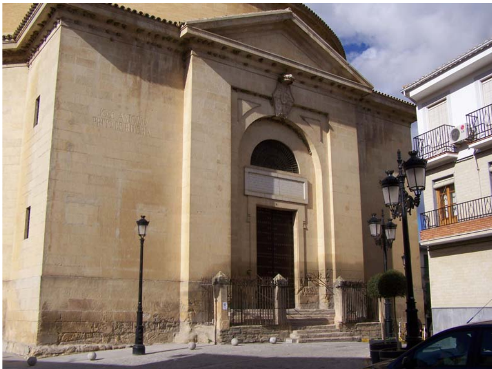
Img. 7: Fachada principal al S-E
